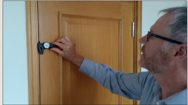
Checking if gaps are uniform and within tolerance.
